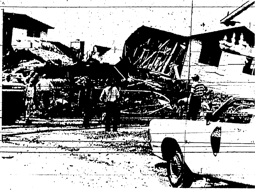
THIS QUAD level home in Denver was blown off its foundation Monday killing Mrs. Mary Ann McGinnis. Officials said a broken gas line possibly caused the explosion. The victim's husband, Michael, was outside the home at the time of the blast and suffered slight injuries. (UPI)
