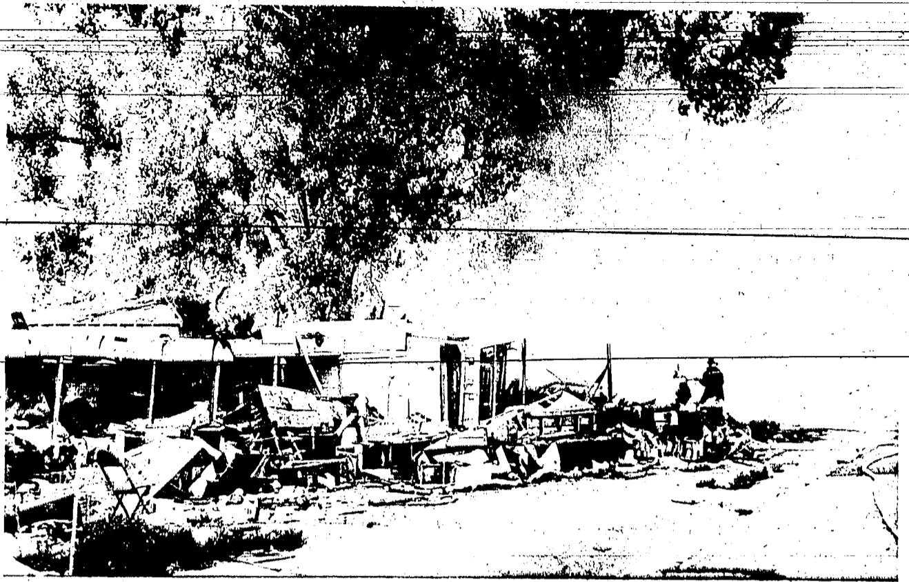
TF shed and other materials destroyed by fire
