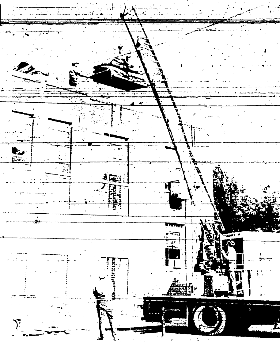
ROOF INSULATION is being lifted to the top of the Jerome County courthouse with a crane operated by Rex Lytle, Lytle Sign Co., Twin Falls. The insulation is being installed as the final step in the addition of a new air conditioning-heating system at the courthouse. Mark Grammer is holding the rope. The work is being done by Clark and Becker, Gooding.
