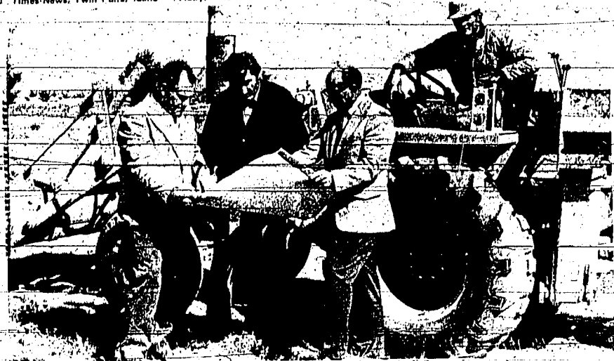
CONSTRUCTION of the new Grace Baptist Church, 789 Eastland Ave. N., began this week. Examining plans prior to starting foundation trenching are (from left) Carl Hoffpau, Dallas, Tex., building consultant; Louie Silman of T & S Construction Co., the contractor; Rev. Robert Seaman, pastor; and Merlin Fairbanks, of Glen Fairbanks and Sons, grading contractor.
