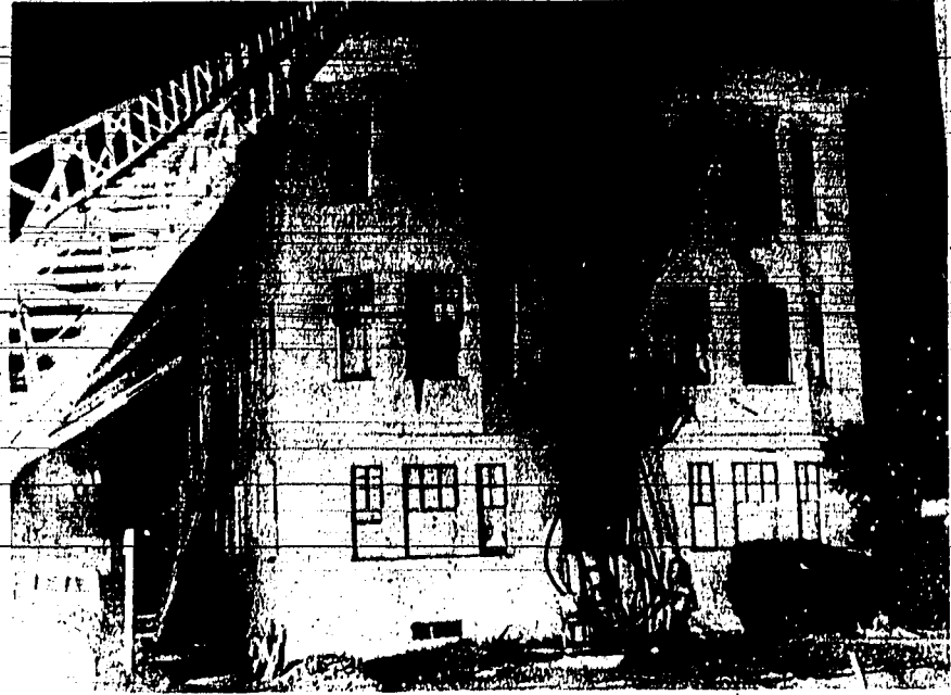
Gutted apartment building in Los Angeles
