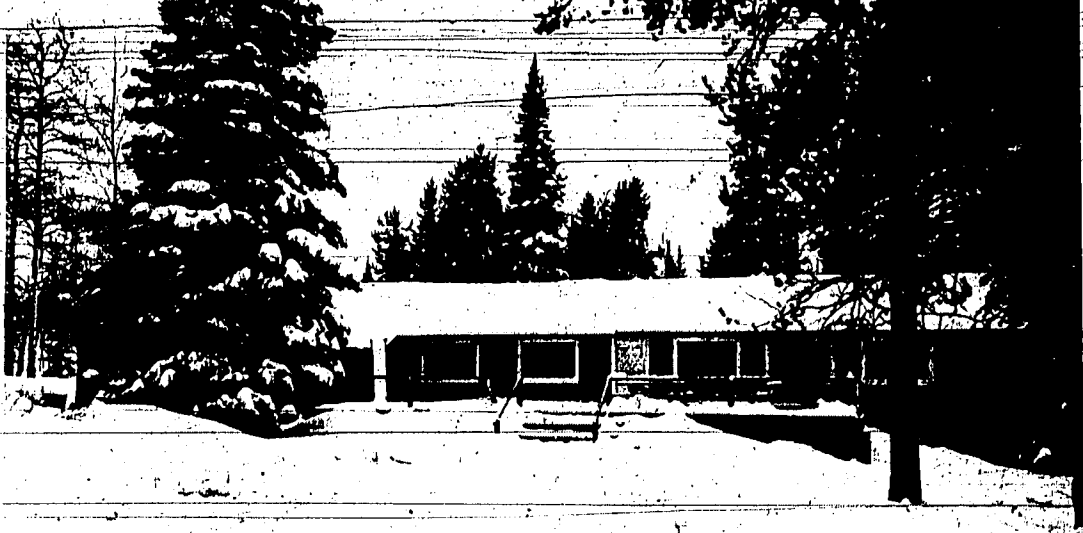
New lodge entrance
