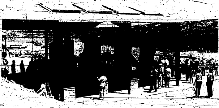
PUMPING STATION on Bell Rapids project is inspected — members of four guests following dedication ceremonies Sunday. Each of three stations has eight 1,500 horsepower pumps with capacity of 9,500 gallons of water per minute for irrigating farmlands. Tour guides were served refreshments during hot, dusty ride at the pumping station.
