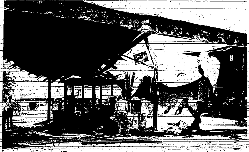
CLEANUP work was underway late Friday and on Saturday at the Don Pieper Gas and Tire Center on Addison Avenue West following a fire at the gasoline pumps. Cause of the fire had not been determined but it destroyed the gasoline pumps, two pickup trucks and considerable merchandise.
