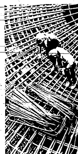
Building reactor WORKMEN build the reactor vessel at the new Colorado Public Service Co. high temperature gas cooled reactor plant at Fort St. Vrain. This type plant is a major user of thorium.
