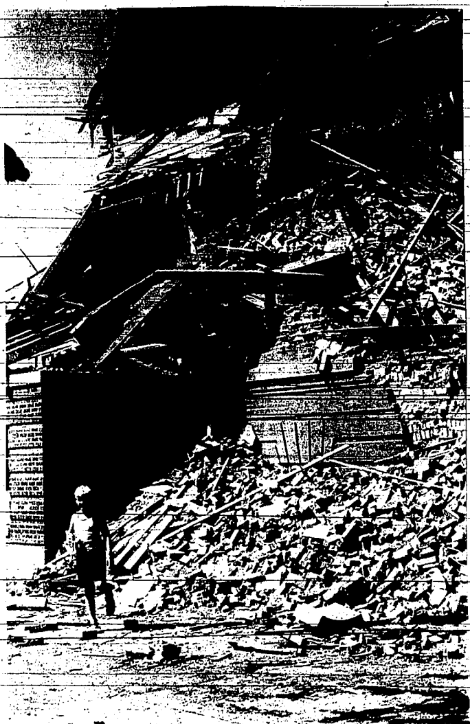
Rubble mounts SMALL boy stands next to giant pile of rubble which was part of the old Lincoln School. Children and adult bystanders were watching Tuesday as wreckers continued demolition of the historic building. The job is set for completion in about three weeks.
