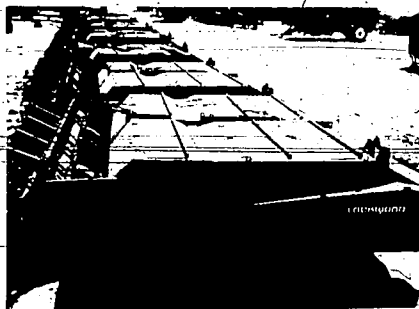
Lockwood Triple Drum Defoliator for efficient beet topping
