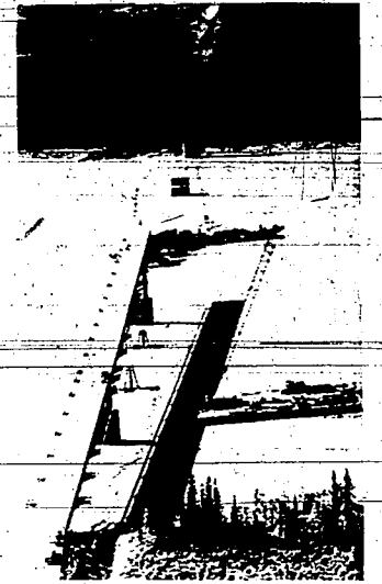
River crossing CONSTRUCTION of the first permanent bridge across the Yukon River in Alaska is proceeding. The span, of which the north end is in the foreground, will link the existing state highway system to the haul road for the Trans-Alaska pipeline. It will also carry the pipeline across the river. UPH
