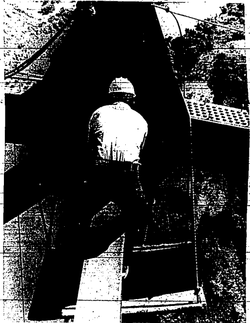
ALLIED Construction Co. engineer Carl Dille "coons" this beam on the new Perrine Bridge. "Cooning" is a term used by ironworkers who routinely walk — and sometimes run — along the beams the way most people would use a sidewalk.
