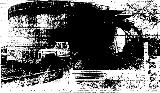
A NEW 300,000-gallon tank for the Jerome City water system located at East 10th Street is nearing completion and expected to be in use in the next 30 days. New booster pumps are being added to the system to improve water pressure.
