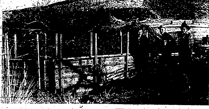
New diversion structure on Rock Creek south of Hansen is nearing completion. It replaces one of several washed out on the creek during all-time record floods last spring.
