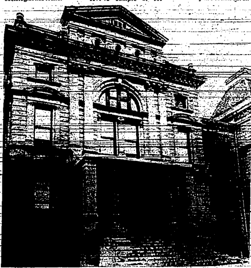
Dudley Gray, a California lawyer who grew up in Iowa, decided the best looking building in the Midwest were the old county seats scattered in the nation's small towns. So, Gray advertised that he wanted to buy a county courthouse and he finally found one for sale. He dismantled the building piece by piece and shipped it to the Los Angeles area to house his law firm. (UPI)
