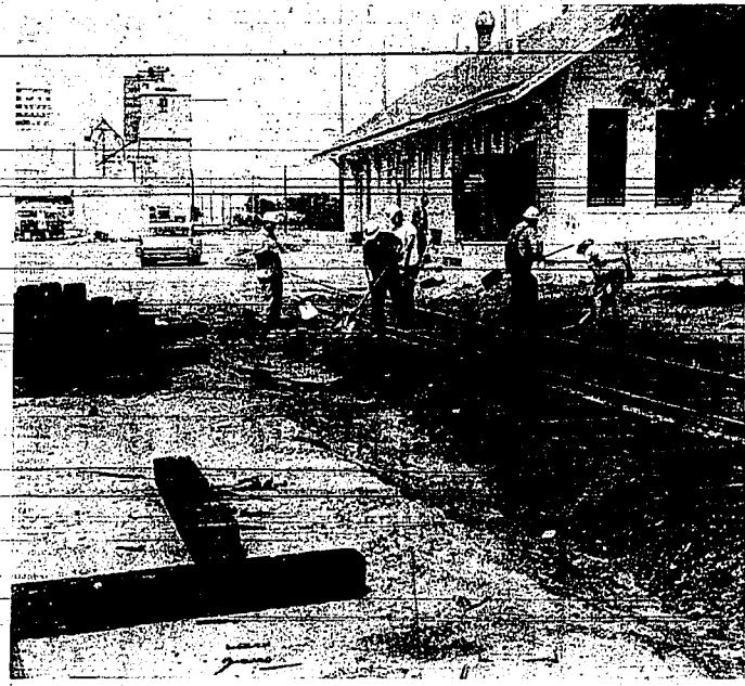
UNION Pacific Railroad workers begin work on a $65,000 project for improvement of the main highway crossing to Rupert. The crews began work Thursday near the depot and southwest of the F Street crossing.
