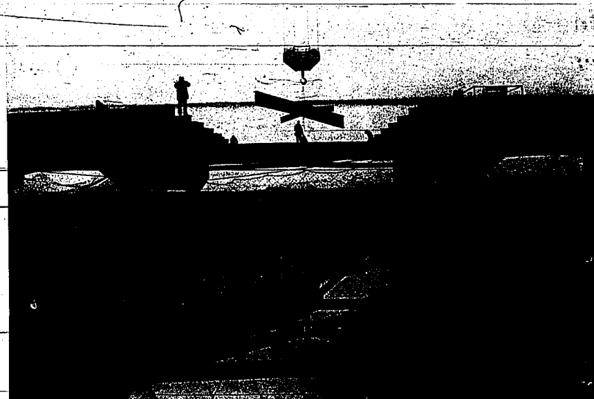
Stringers were carried into position by cableway hook on the new bridge
