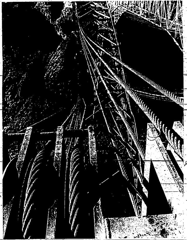
50-ton jacks support the weight of the north arch prior to the closing of the arch.
