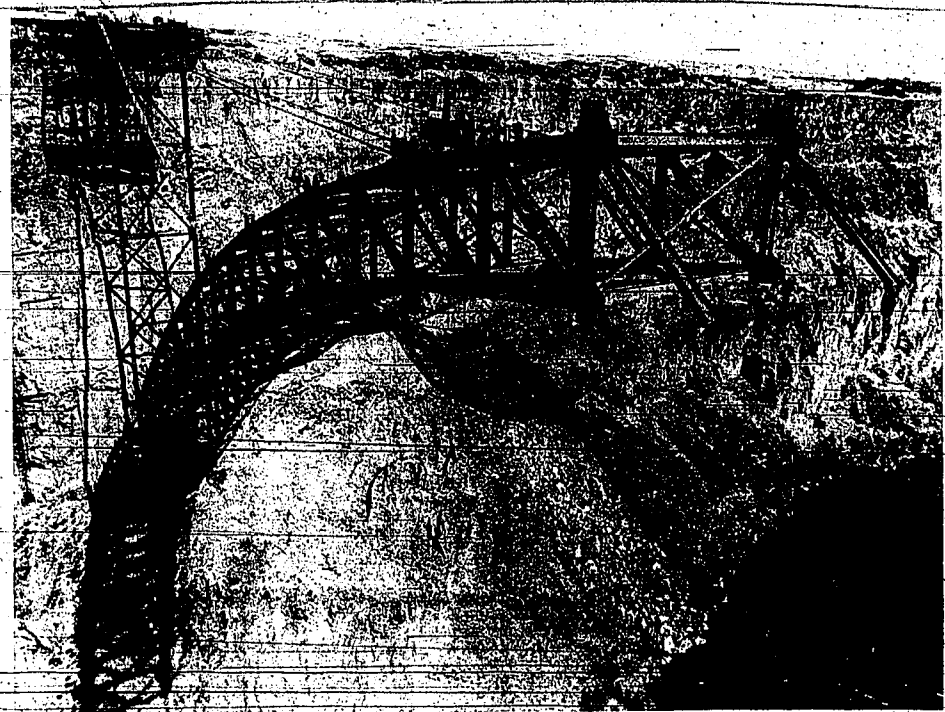
The north arch thrusts itself over the canyon to meet the south arch.
