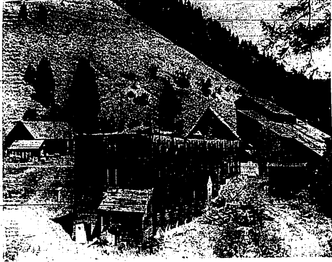
Buildings in ruin
