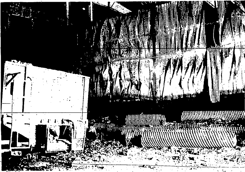
Tattered insulation after fire in Jerome spud cellar
