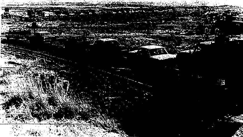
CARS and trucks were sitting out along US 93 and the Idaho 21 cutoff to Jerome as drivers waited for blasting along the road project north of the newly opened four lane rim-to-rim bridge.
