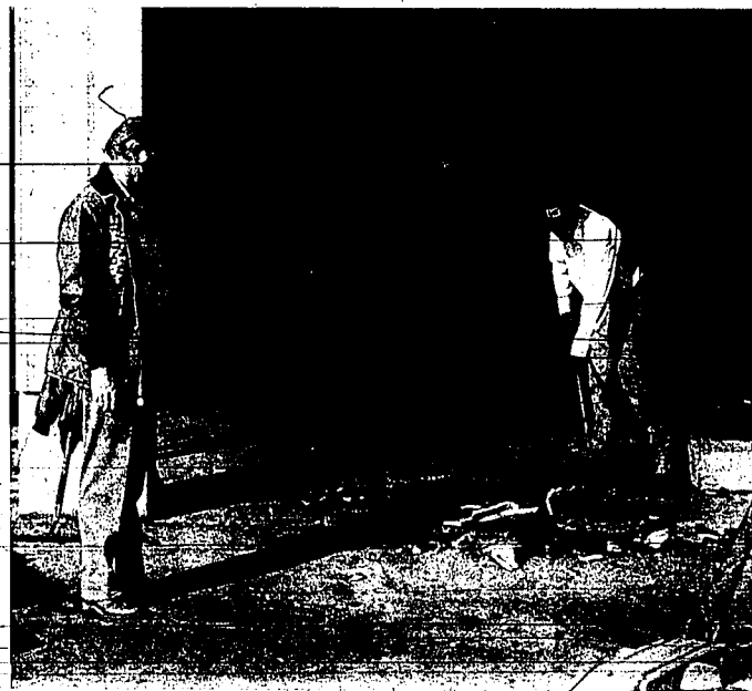
ACE HANSEN, owner of a car dealership at 1654 Blue Lakes Blvd. N., which was almost completely destroyed by fire Tuesday, watches as one of his employes pushes debris out of a smoke-blackened garage.
