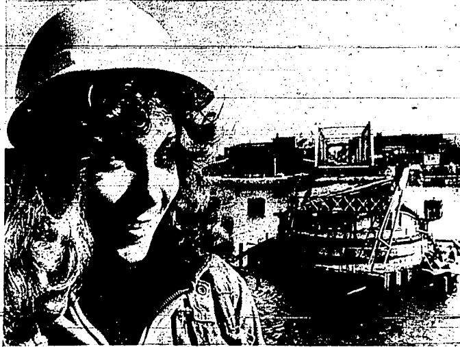
THE JOB market for 18-year-old high school graduate Wendy Dore was slim up until a month ago. After studying to be a secretary, and finding no jobs available, Wendy became a laborer with a wrecking company now in process of dismantling the Third Street Bridge, Bay City, Mich. She does the same work as the men on the project including operating the 90-pound jackhammer and cutting torch. (UPI)
