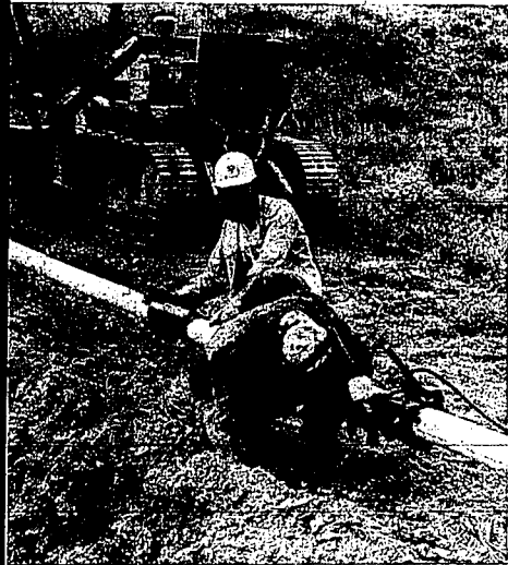
WELDER, Ed Wickham, Hagerman, joins two sections of water line on lower slopes at Solder Mountain where work is underway on the final stages of a new snow making system. Dave Wheeler, resort manager, holds line in place. This branch line will provide water for snow making along the J-bar lift, one of several slopes to be served by the system.
