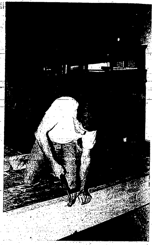
WORK HAS BEGUN TO RESTORE TO AN ENGLISH COLONIAL ... Stan Rose, owner, may open the house to tours
