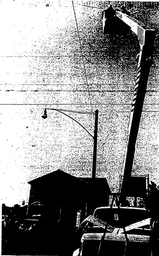
UTILITY TRUCKS LIFTED POWER LINES AND REMOVED LIGHTS A police escort directed traffic for Bruce Miller-Movers
