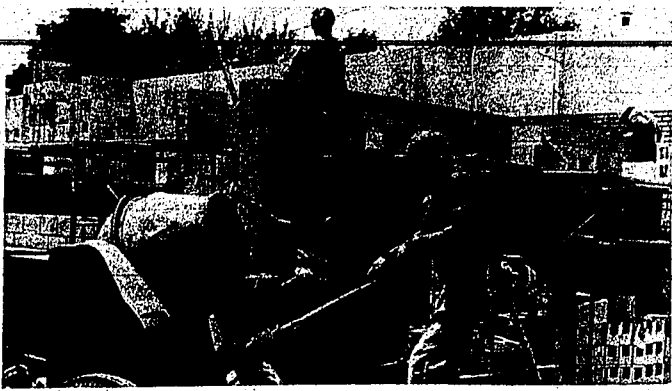
A $41,193 addition is under construction at the Gooding county courthouse. Contractor for the project is Marvin Pierson, Gooding. County Clerk Margaret Clements said the new structure will be used to house records for all departments. It is located next to the clerk's office.
