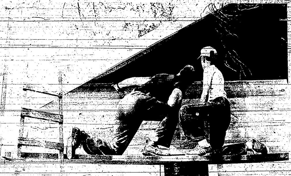
GETTING SIDING TO FIT TAKES SPECIAL ATTENTION Methodists put siding on infirmary at Camp Sawtooth
