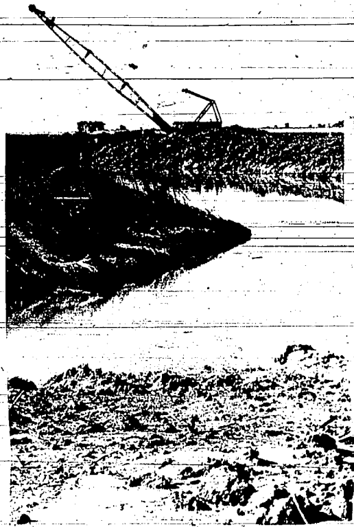
THE FISH and Game Department hired the drag line pictured above to dig channels in the bottom of Carey Lake to help fish survive through the hard winters. The channelization will also create islands like the one at left to aid waterfowl nesting and dikes like the one at the right to facilitate hunter access.
