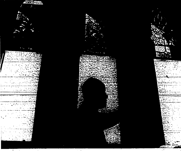
In Denver PASTOR Henry Kelly is silhouetted in gaping hole where stained glass windows were stolen from his church. Kelly says he plans to replace the stained glass with regular glass because of the high expense. Six windows valued at $1,200 were stolen.
