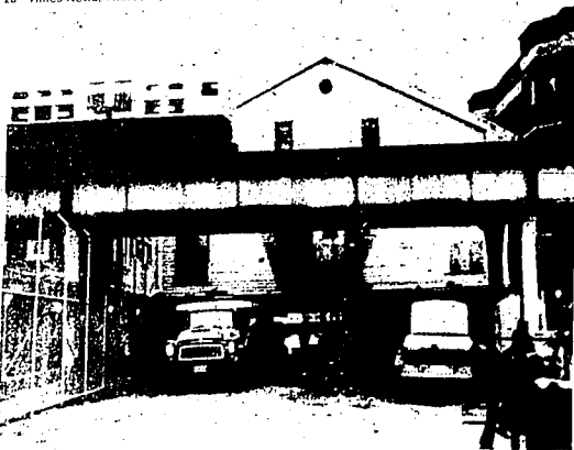
ELEVATED RAILWAY tracks halted the movement of Chicago's oldest house to a new site two miles away. The moving crew will raise the house above the level of the tracks, winch it across, lower it, and continue the trip. Built in 1836, the house will be restored at its new site.
