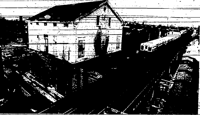
JACKS MAKE — a high rise as they raise the Henry B. Clarke house, oldest house in Chicago, 25 feet above ground — to enable movers to ease it over the Chicago Transit Authority tracks this week.
