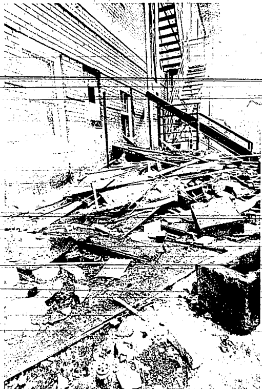
DEMOLITION — OF — the abandoned Lincoln School on Third Avenue West in Jerome began last week. Work is progressing rapidly and the school district plans to auction salvaged materials. Demolition of the 65-year-old building will provide playground space.
