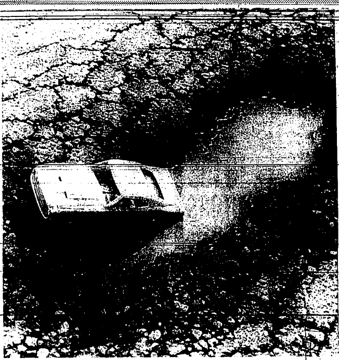
HIGHWAY CHUCKHOLES CAN BE HAZARDOUS TO YOUR HEALTH—... this year the holes are exceptionally large and plentiful on Idaho highways
