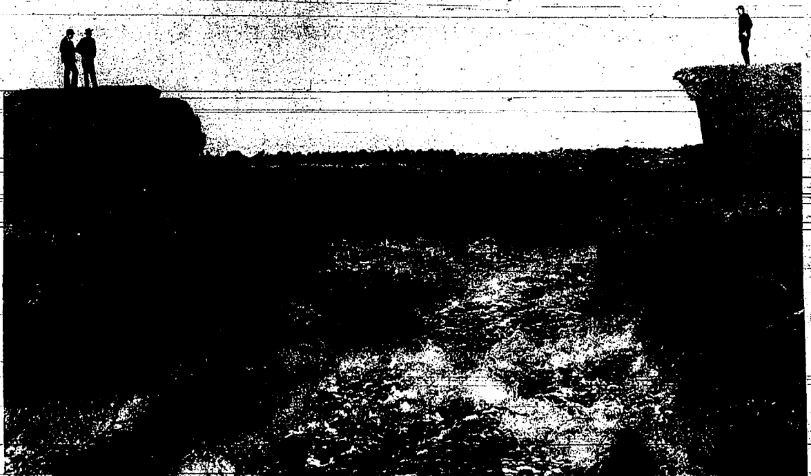
TWIN FALLS CANAL CO. OFFICIALS LOOK OVER 80 FOOT GAP IN HIGH LINE CANAL WALL
