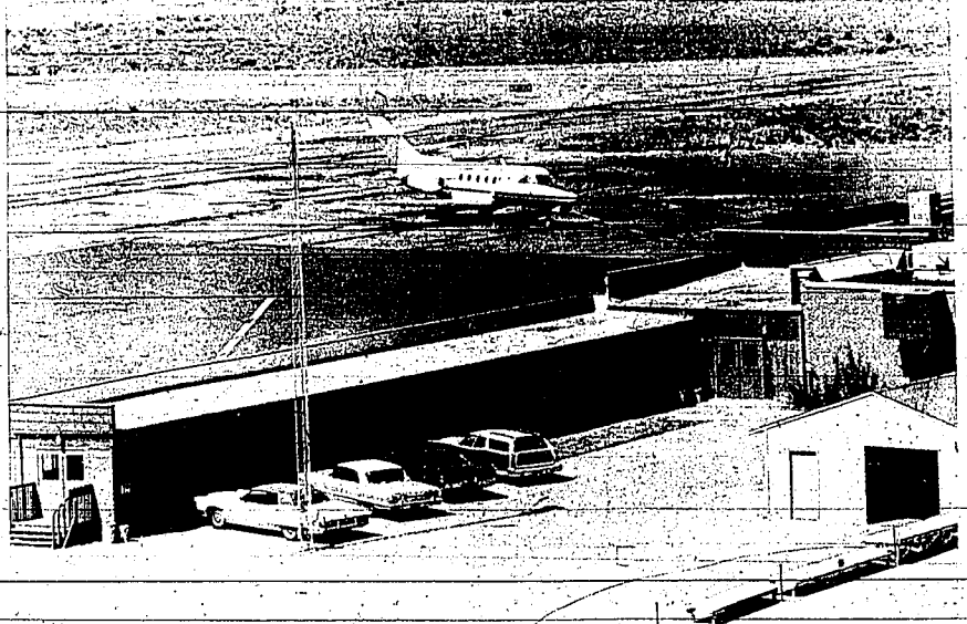
EXTENSIVE IMPROVEMENT TALKED ABOUT FOR TWIN FALLS' JOSLIN FIELD ... majority of traffic at the local airport is privately-owned airplanes
