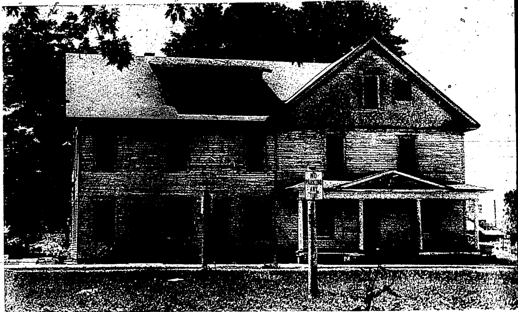
FILER'S ONLY THREE-STORY BUILDING, A HOTEL SINCE 1908, HAS NEW ROLE ... It's 11 rooms, five apartments are now home for Marti Nowak and family
