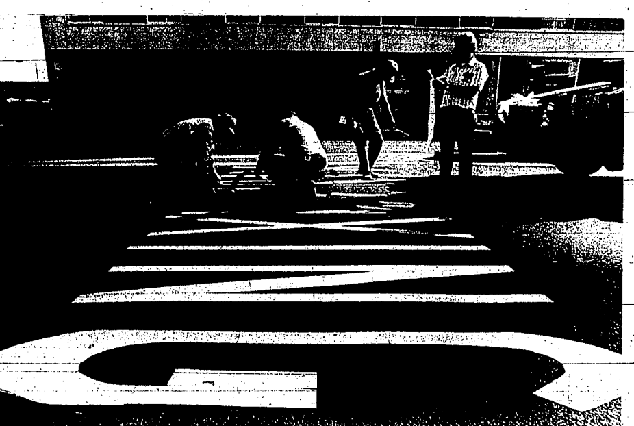
In a safety improvement plan at Main and Shoshone, city workers lay pedestrian crossing warnings
