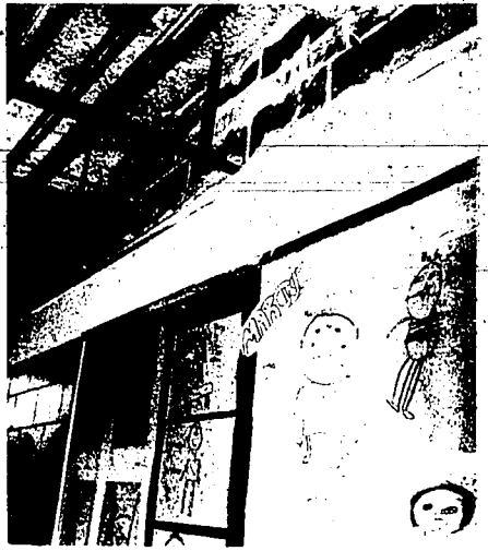
Asbestos insulation is exposed in school ceiling.
