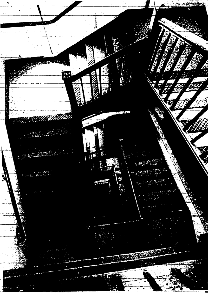
One of two emergency exit stairwells added to Providence College's Aquinas Hall since last year's tragic fire
