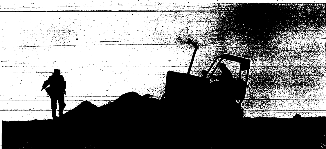
Paul Wilka, left, and Ray Simpson filled in main break on Highline canal Tuesday
