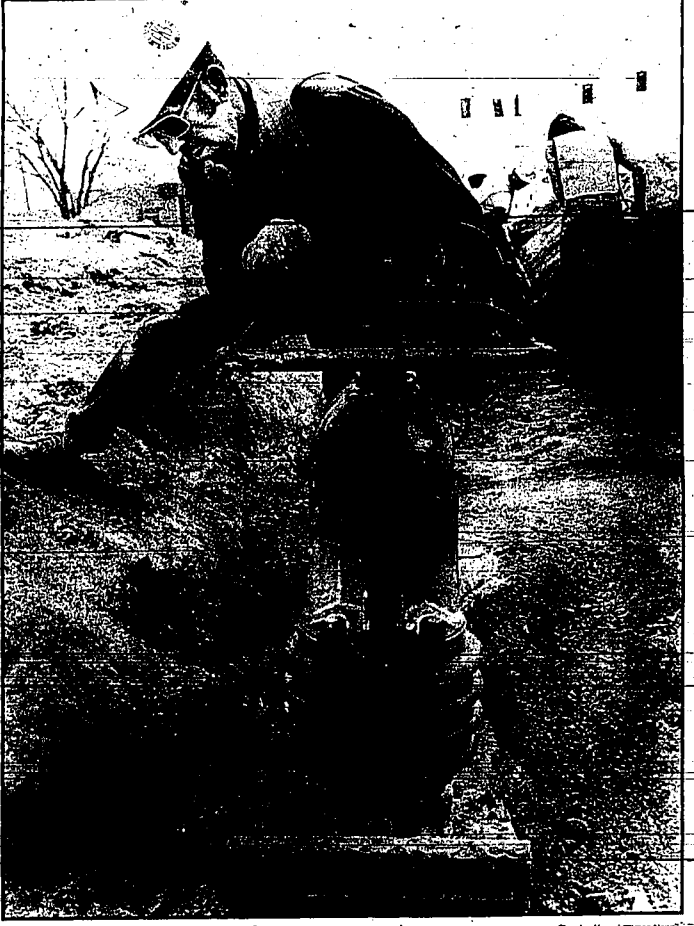
Foot comes in handy Frank Vigil's job Monday on the reconstruction of Addison Avenue in Twin Falls was to run a power tamper over a trench being filled in. The big, weighted foot of the tamper compacts the loose dirt around new pipe, but Vigil's foot helped him keep the machine on course.
