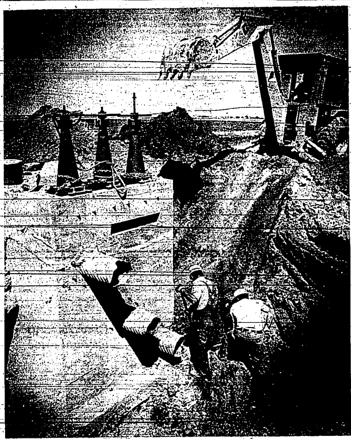
Rupert water department workers dig around diversion unit looking for leaks in the outlet pipes. Diane Hagaman/Times News
