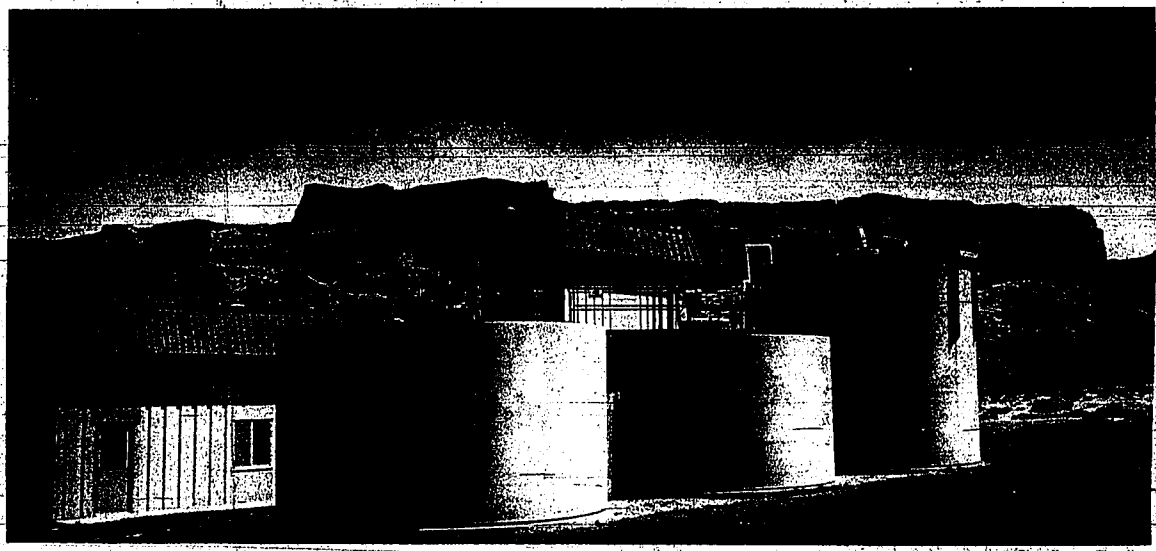
While Twin Falls city officials seek private land for dumping sludge, the treated waste is stored in these tanks near the sewage treatment plant.
