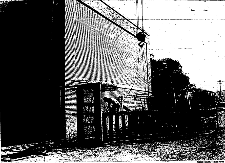
Fire escapes recycled
