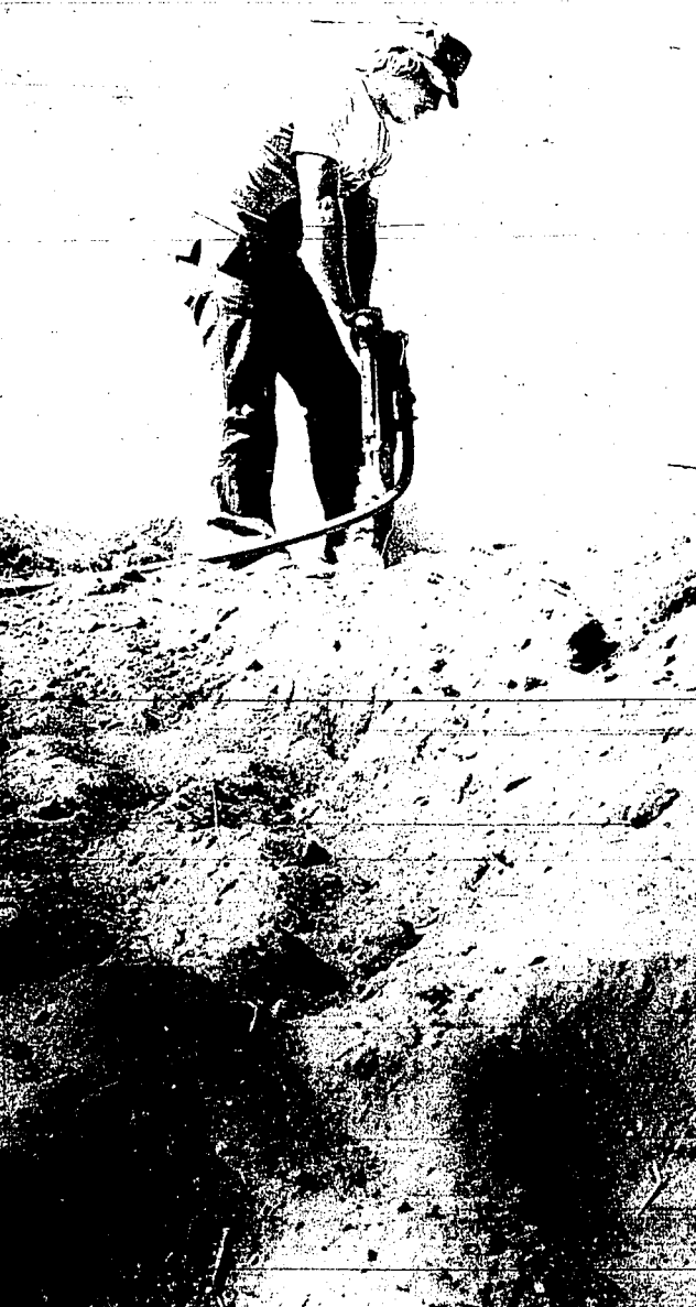
Steve Troubridge blasts away at lava rock where Jerome's new sewer lagoon building will stand
