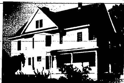
Originally the Ostrander home, this house was the Crabtree motel
