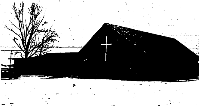
St. Paul's Lutheran Church's new facilities, built largely by congregation members
