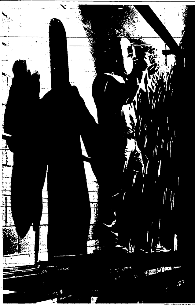
A welder, with a little help from his shadow, welds a heat line for the new Paul Elementary School
