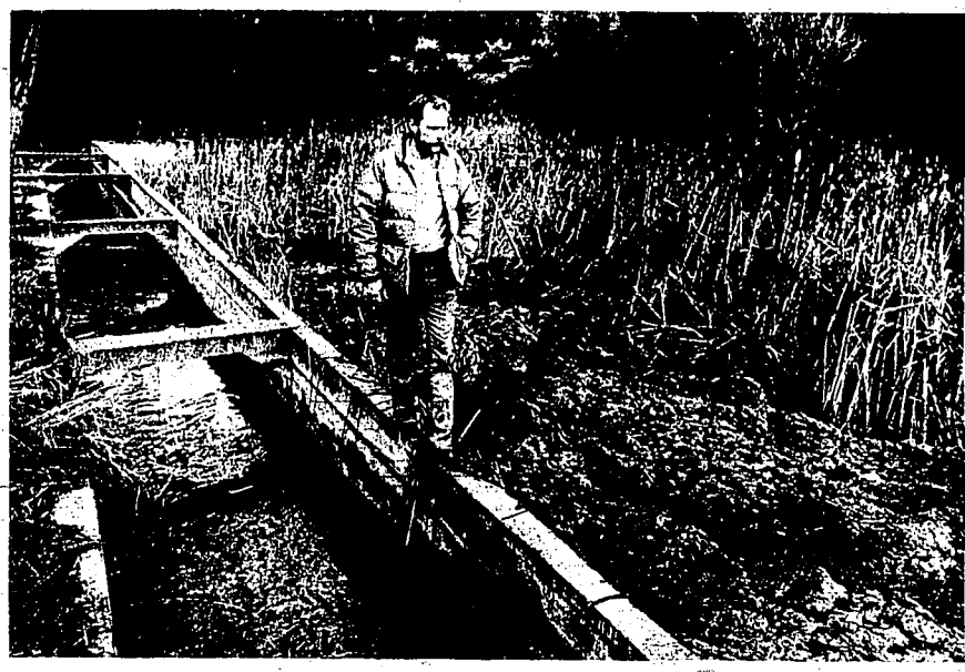
Bruhn inspects site where 12 new raceways of a proposed 60 additional will be built at the Hagerman hatchery
