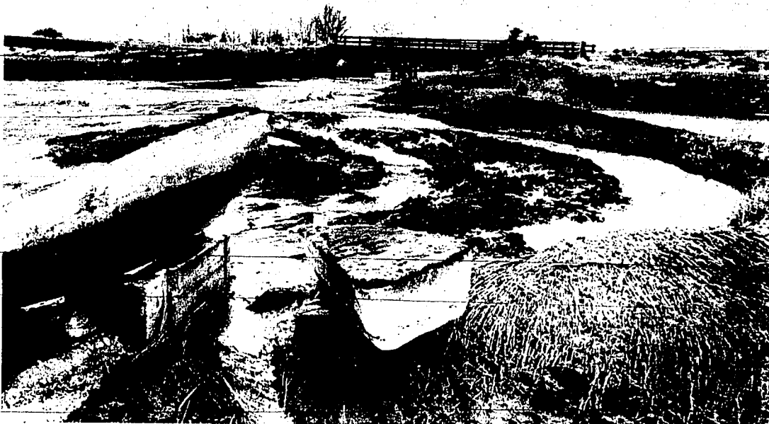
Large chunks of ice floating down the swollen Little Wood River Tuesday damaged a bridge on U.S. 93 northeast of Shoshone.
