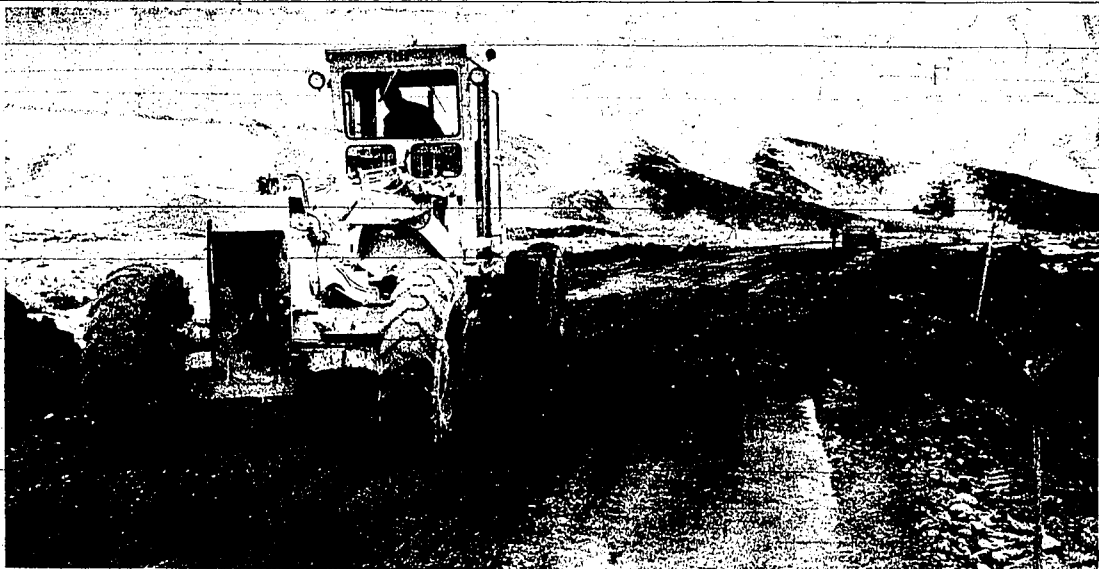
Although still very rough in spots, highway crews worked all day Wednesday to make the road passable between Carey and Arco after storm damage Tuesday.
